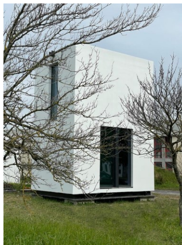
Figure 20. Pilot Construction – LNEC Campus.
