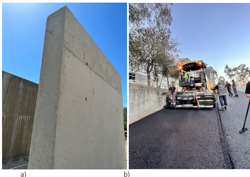
Figure 1 – a) reinforced concrete wall with RCA; b) experimental section of bituminous mixtures with RCA
