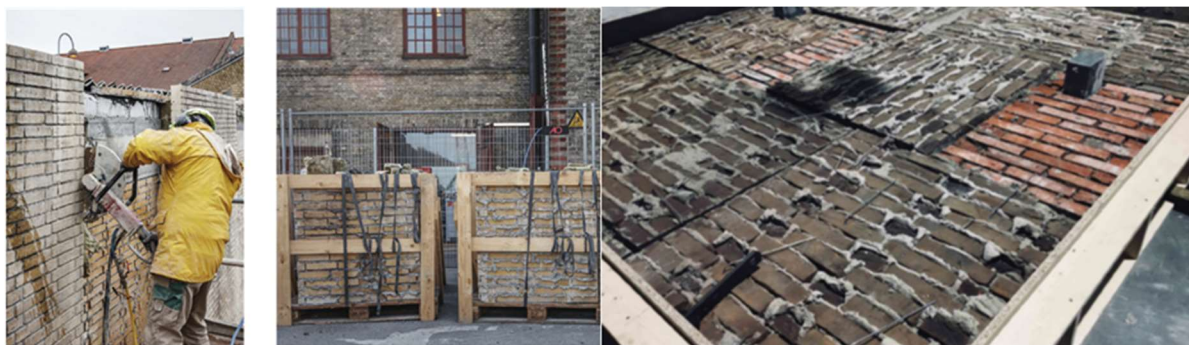
Figure 16 - Steps in preparation of the facade module (cutting from existing building, transport to the site, installation in steel frame) [22].
